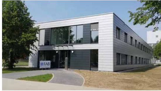
Fig. 6.10: New office Building at the X-FAB site in Itzehoe (Germany)
