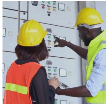
Industrial power supply
