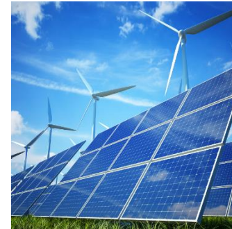
Renewable energy generation
